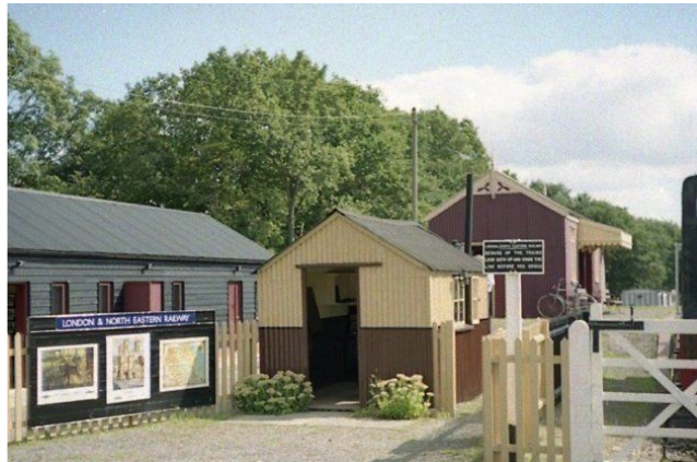
Wilby Station Hut: restored and in its new position (photo: Mid-Suffolk Light Railway)
